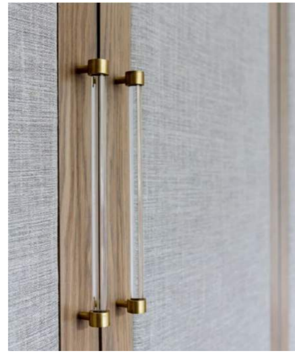
Timber frame & Fabric inserts
